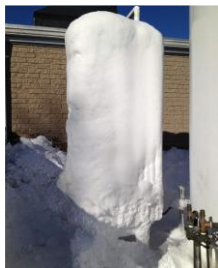
Gas withdrawal exceeding vaporiser capacity
