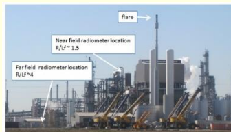
Figure 1: Overview of hydrogen plant, & flare highlighting near and far field data collection locations.
