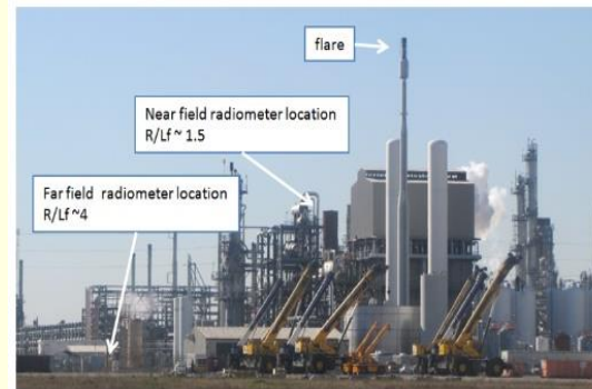
Figure 1. Overview of hydrogen plant, & flare highlighting near and far field data collection locations.
